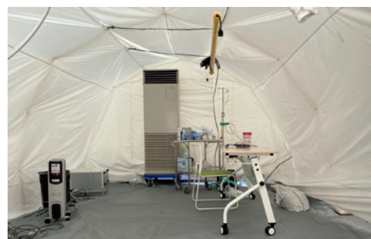
The tent's interior is equipped with a negative pressure filter system to prevent the outflow of the virus. It is used for PCR tests for COVID-19.
