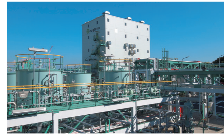
Euglena Co., Ltd.'s biofuel production plant will be fully operational in 2020, after completing a two-year trial.
