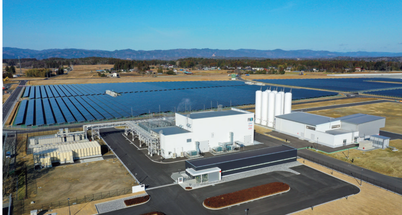
The world's largest facility for producing hydrogen using renewable energy is the Fukushima Hydrogen Energy Research Field (FH2R).
