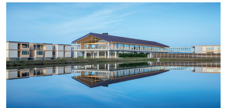
The Shonai Hotel Suiden Terrasse, built from wood, was designed by the prominent Japanese architect BAN Shigeru. Suiden means paddy, or rice field. The hotel, built to look as if it is floating amidst rice paddies, is a new attraction that adds to the appeal of Tsuruoka City.
