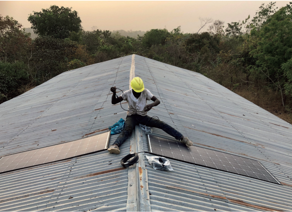
The solar sheets designed by Kawaguchi Steel can be installed on tin roofs because of their light weight. Before the school had electricity, all the classrooms were dark, and on cloudy days, classes were sometimes even held outside.
