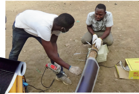
Pictured left is a flexible solar sheet. Streetlights with such sheets wrapped around their poles not only introduce light to areas that previously lacked electricity, but also play a part in improving security there.
