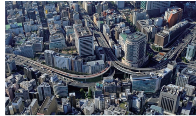
Japan’s Metropolitan Expressway has many curves and junctions, demanding different capabilities from automated driving technology than most expressways in Europe and the U.S.
