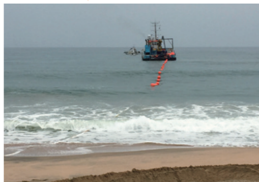
Cable to Angola during marine installation.
