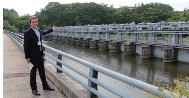
Joost standing in front of the Jurokkyo Sluice Gate, a key component of the Asaka Canal construction project. It regulates the water level of Lake Inawashiro while allowing water to flow to the Asaka Plains.
