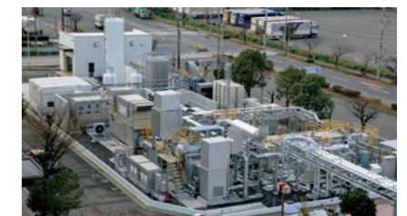
A system for supplying hydrogen will not have an impact unless demand is also stimulated. In April 2018, in Port Island of Kobe City, Kawasaki Heavy Industries, Ltd. and Obayashi Corporation successfully conducted the world's first demonstration of supplying heat and electricity in the urban area using a gas turbine fueled by 100% hydrogen.
