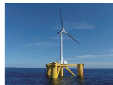
A 7-megawatt floating wind turbine has been constructed off the coast of Fukushima under a project commissioned by the Ministry of Economy, Trade and Industry. The blades reach a height of 200 meters (about 660 feet) above the ocean. Photo: Fukushima Offshore Wind Consortium.
