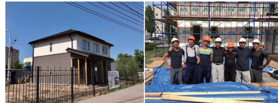
Four Japanese contractors (white helmets) have been dispatched along with the necessary construction materials. A total of eight Japanese and Russian contractors worked on the construction during the short span of three months from laying the foundation to finishing the outer walls. The team worked closely together, and the Russian team members have learned very quickly about the Japanese styles of housing construction.
