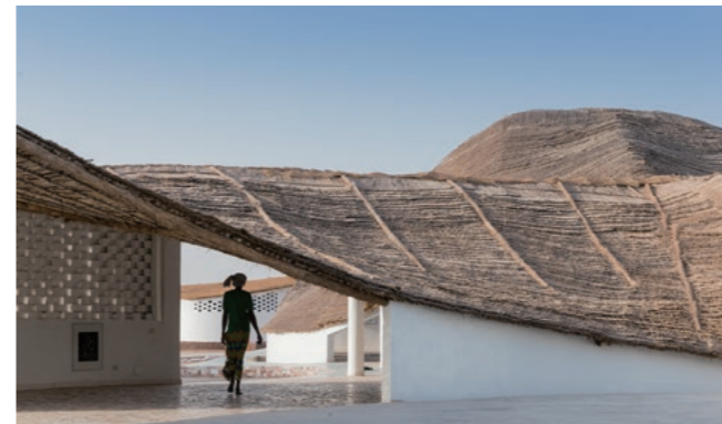
Constructed with a thatched roof, sun dried mud bricks and bamboo, the center was built with local materials and labor. Its defining characteristic of a steep thatched roof harvests rainwater that serves nearly 30% of the village's household needs. © Iwan Baan
