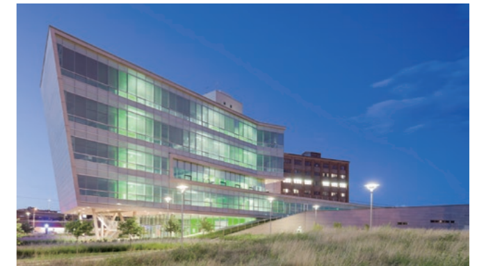
The building houses a collaborative federation of experts on environmental research such as chemistry, engineering, material science, psychology, and thermodynamics. Topics such as strategies for energy efficiency, indoor environmental quality and site remediation techniques were discussed throughout the project. © Iwan Baan
