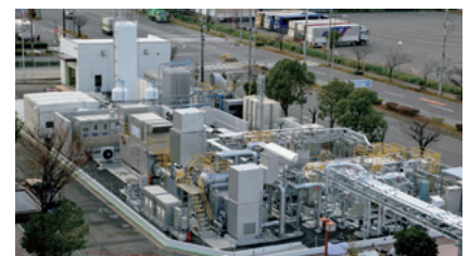
A system for supplying hydrogen will not have an impact unless demand is also stimulated. In April 2018, in Port Island of Kobe City, Kawasaki Heavy Industries, Ltd. and Obayashi Corporation successfully conducted the world's first demonstration of supplying heat and electricity in the urban area using a gas turbine fueled by 100% hydrogen.
