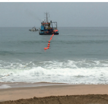
Cable to Angola during marine installation.
