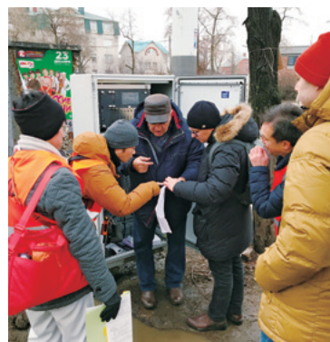
Although this was Kyosan’s first project for Russia, the company was able to overcome issues in adapting the system through trial and error together with its Russian counterparts.
