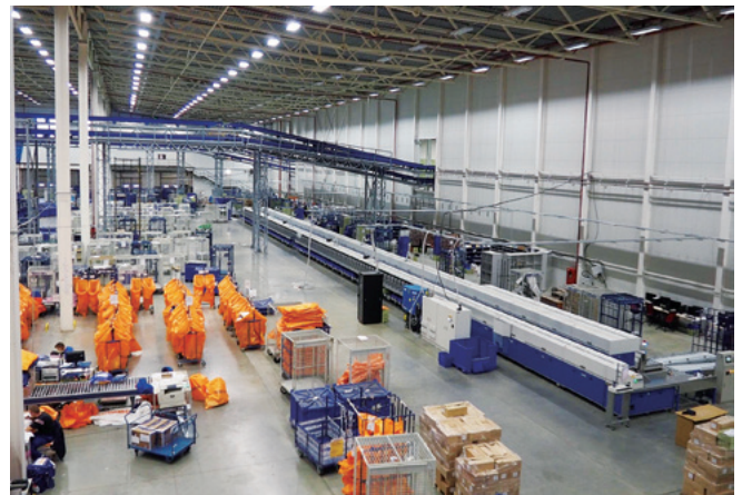
Russian Post’s Vnukovo Logistics Center is an enormous facility equivalent to about six gymnasiums in scale. Using conveyor belts to reduce the burden on the facility’s staff was one of the approaches used by Toshiba.
