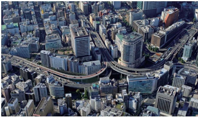
Japan's Metropolitan Expressway has many curves and junctions, demanding different capabilities from automated driving technology than most expressways in Europe and the U.S.
