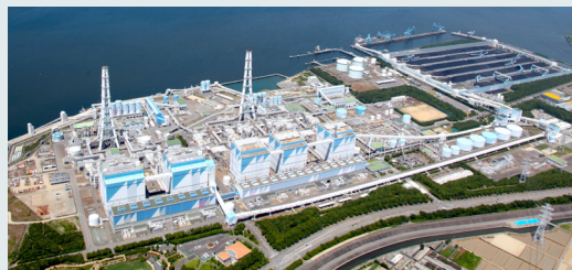
Several MOUs on the production and utilization of ammonia were signed at the AZEC Public-Private Investment Forum held in March 2023. The photo shows the Hekinan Thermal Power Station in Aichi, where a demonstration project to generate electricity by co-firing ammonia and coal is underway. JERA CO., INC.
