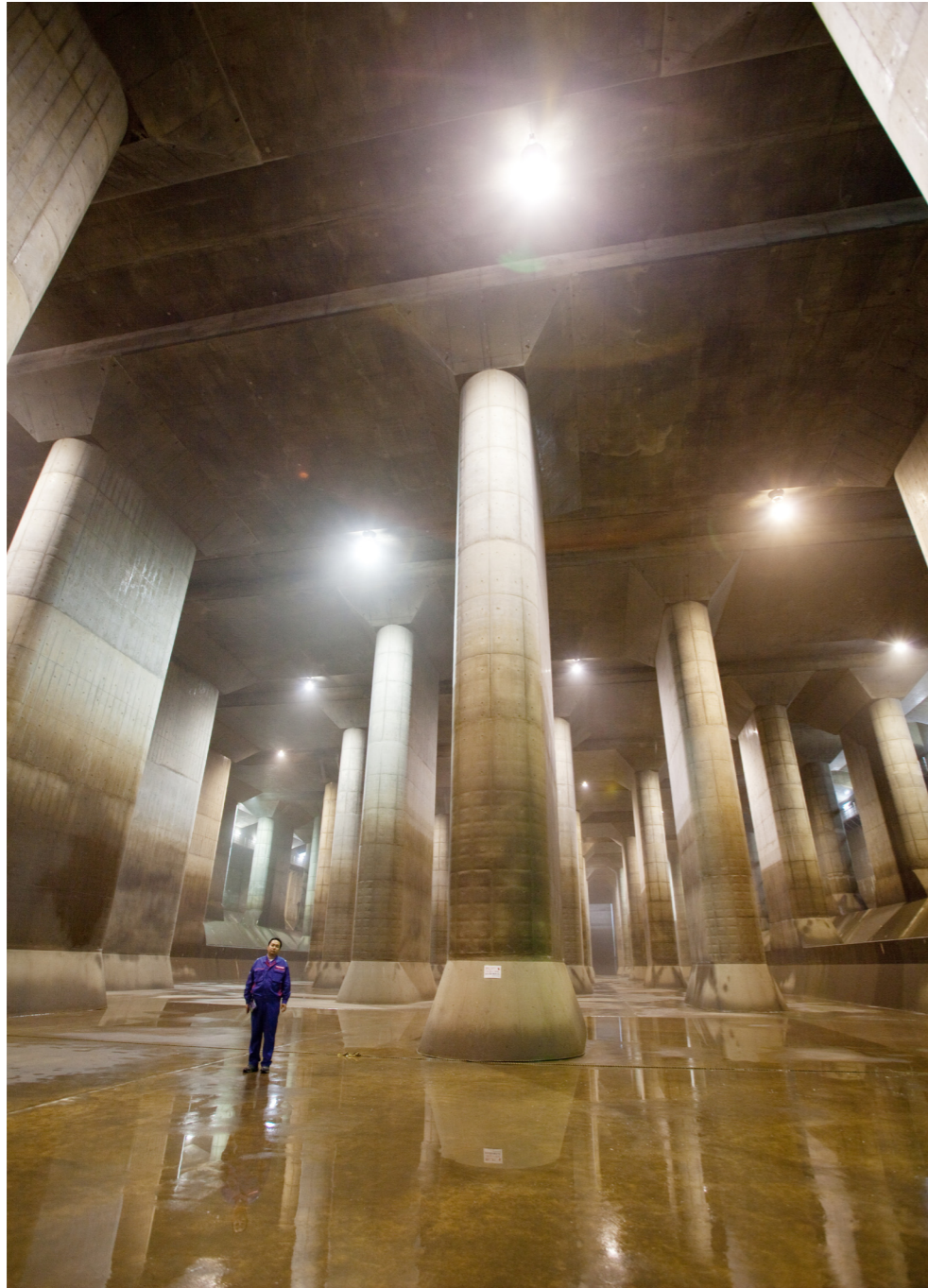
Inside of the pressure-adjusting water tank of the Metropolitan Area Outer Underground Discharge Channel.
