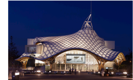
One of Ban's most important works: the Centre Pompidou-Metz, a provincial branch of the Centre Pompidou built in 2010. Its roof is made of wood and features beautiful organic curves (photo by Didier Boy de la Tour).
