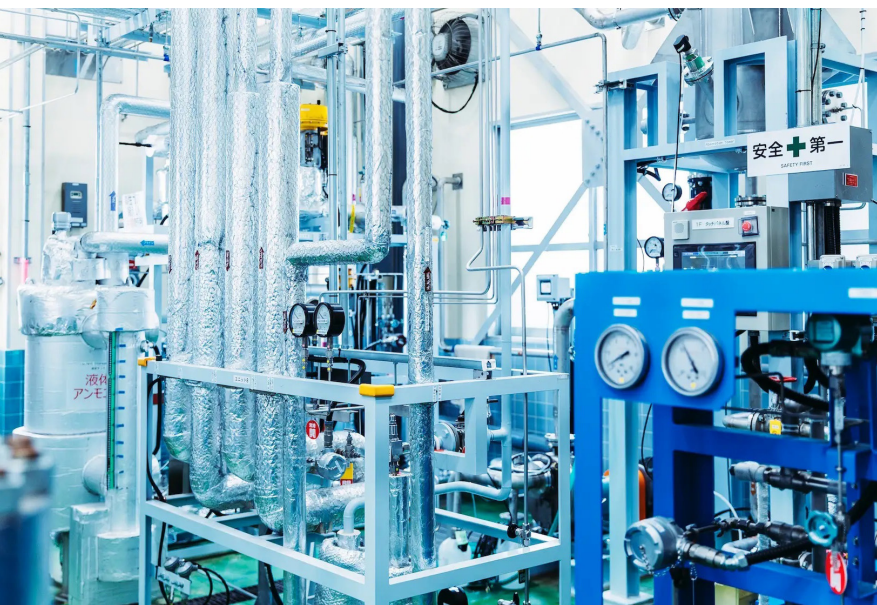
Top: Ajinomoto Co., Inc., a Japanese food company and Tsubame BHB shareholder, made its factory in Kawasaki City available for the installation of the startup's pilot plant. In operation since 2019, the plant produces 20 tons of ammonia a year at a steady pace.
