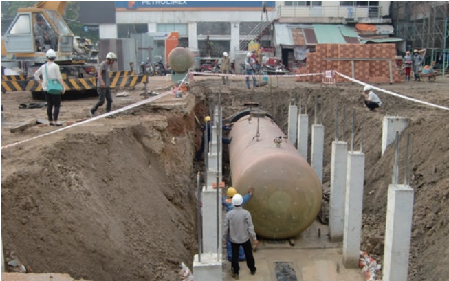
A double-wall tank made in Vietnam is laid in the ground at a gas station in Ho Chi Minh City.
