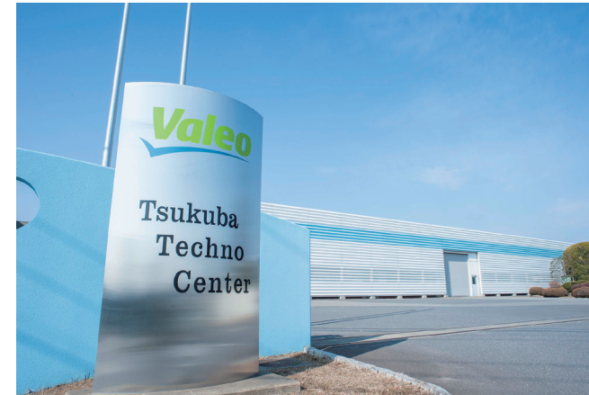
Tsukuba Techno Center in Tsukuba Science City, 50 km northeast of Tokyo. Since self-driving automobiles require highly confidential technology development, Valeo built an exclusive test track.
