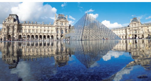
Photocatalysis acts as an antifouling and antifogging effect simply by the irradiation of light. It has also been used in the glass covering the pyramid-shaped entrance of the Louvre Museum. The glass maintains its transparent beauty by decomposing dirt.
