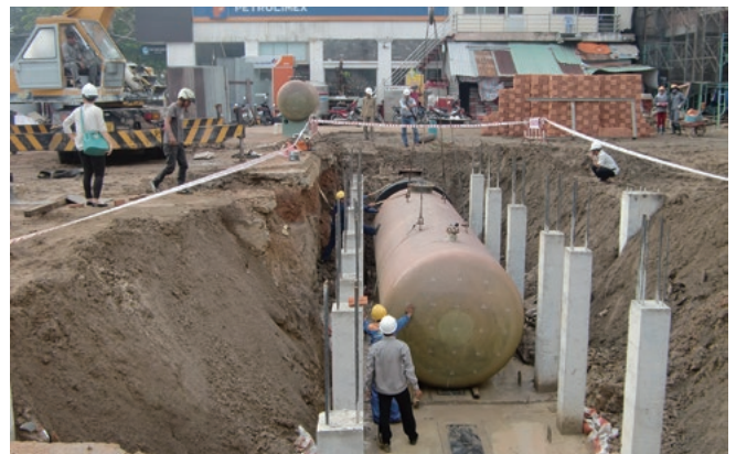
A double-wall tank made in Vietnam is laid in the ground at a gas station in Ho Chi Minh City.
