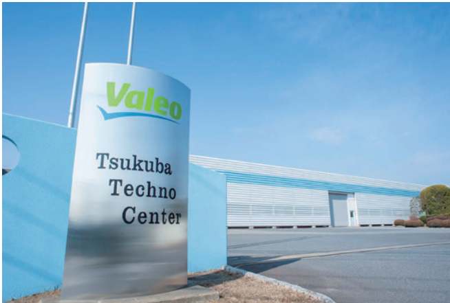
Tsukuba Techno Center in Tsukuba Science City, 50 km northeast of Tokyo. Since self-driving automobiles require highly confidential technology development, Valeo built an exclusive test track.
