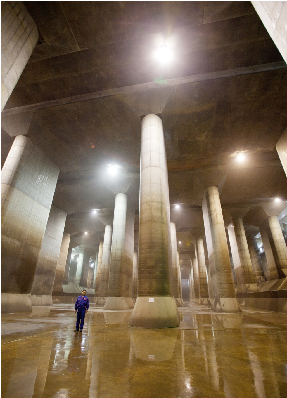
Inside of the pressure-adjusting water tank of the Metropolitan Area Outer Underground Discharge Channel.
