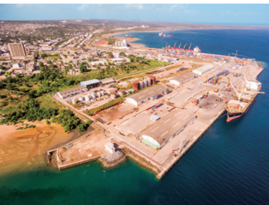
The establishment of a container yard is also planned in this renovation project. Serving as a gateway, Nacala Port is expected to lead to economic development of the surrounding area.
