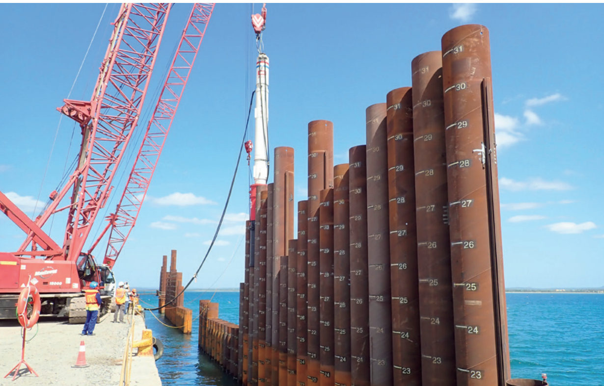
Driving in of steel pipe sheet piles at Nacala Port for new quay construction. Large cargo vessels will be able to enter the port, bolstering the sea transport capacity of northern Mozambique.
