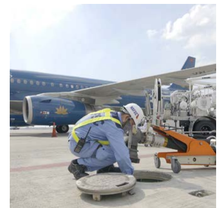
Hydrant method that allows safe refueling with a large volume of aviation fuel delivered in a short period of time.
