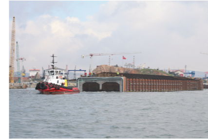
1. Tunnel construction barges floating in the Bosphorus, with the First Bosphorus Bridge in the background. 2. Large concrete tunnel sections for the undersea portion were towed to the site by tugs. 3. Bosphorus Strait tunnel route map and cross-section view.
