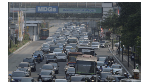
A Jakarta street earmarked for the laying of new underground sewerage pipes. Consistently heavy traffic means the road cannot be closed for the necessary construction work to take place.
